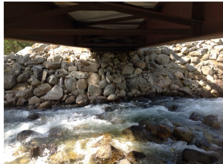
Right Bank Abutment when facing downstream
