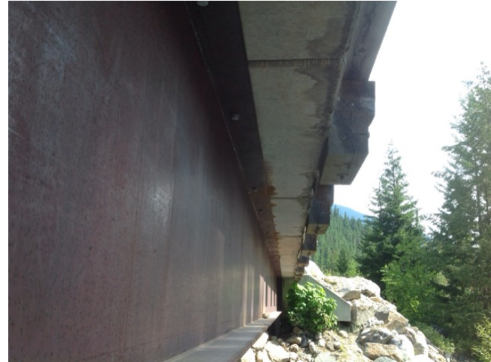
girder to deck connection
