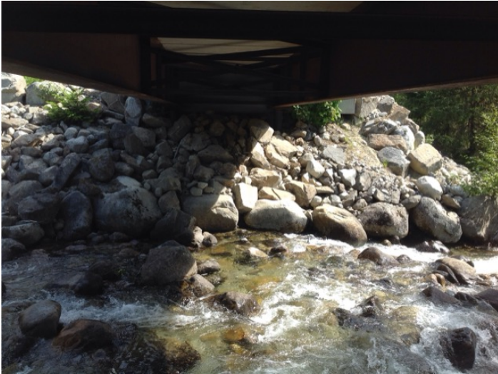
Left Bank Abutment when facing downstream
